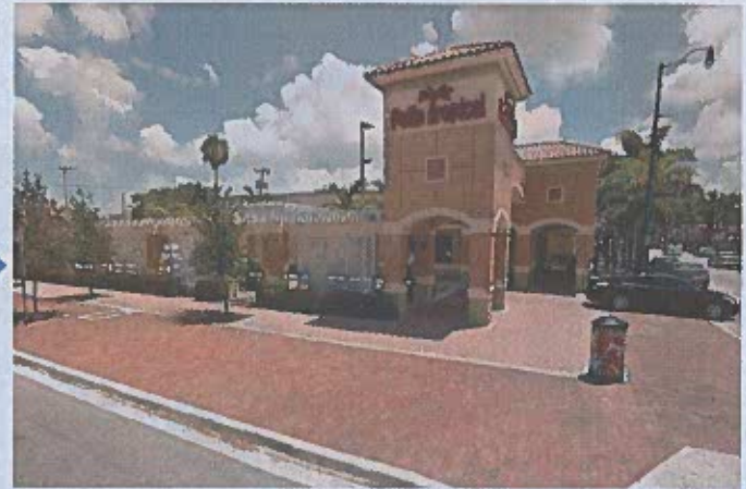
Form Based Code: A Pollo Tropical (fast-food restaurant) in Miami, FL. Parking is hidden by pergola, wide sidewalks, sign on a tower.
